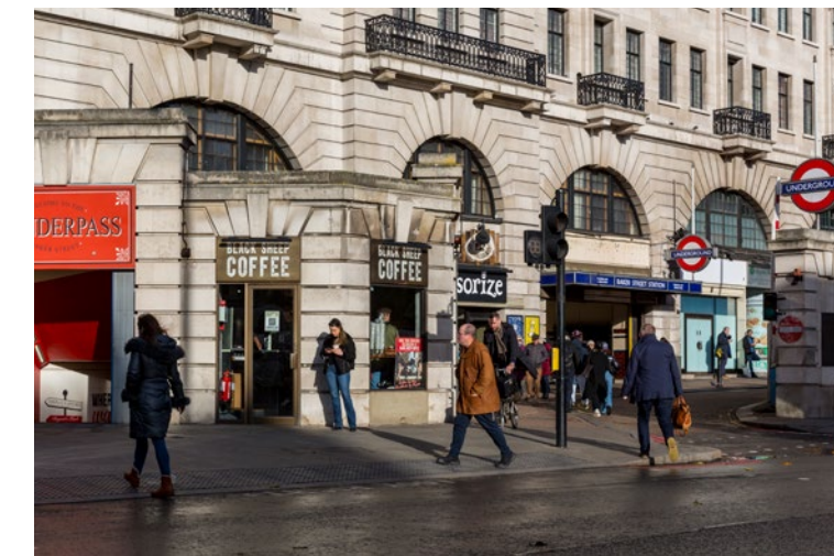
Energy Performance Certificates for all properties to build a carbon emissions baseline
