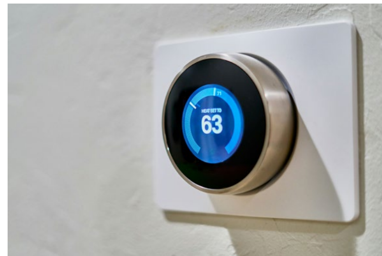
Smart meters are being installed to help our tenants with consumption
